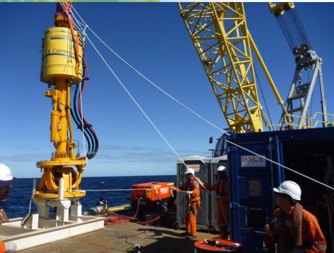
CETO3 pump, attachment & connector installation
