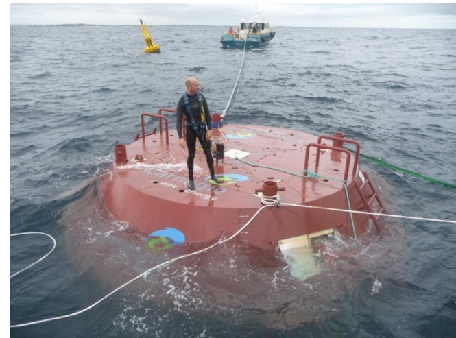
Buoyant Actuator installation
